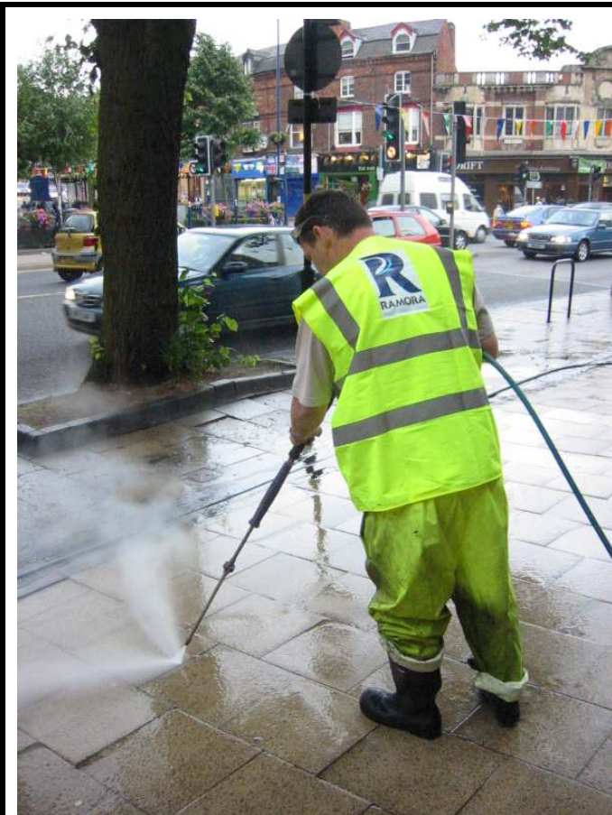
Jet blasting the pavements of Moseley shopping centre in preparation for the judging day for Moseley in Bloom
