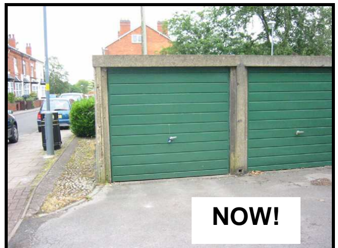
Council owned garage door in Middleton Road earlier this year
